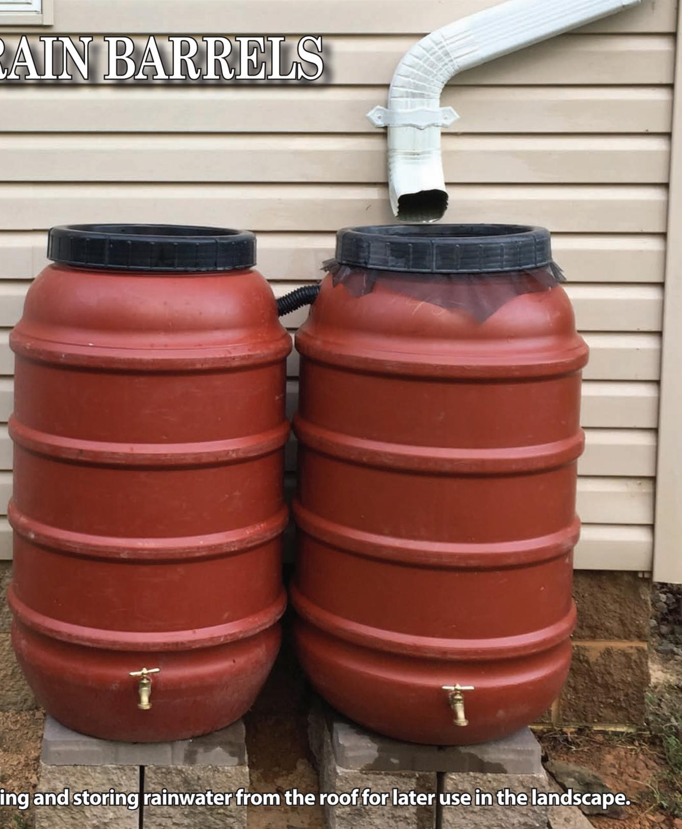
**Rain barrels reduce runoff by capturing and storing rainwater from the roof for later use in the landscape.**
